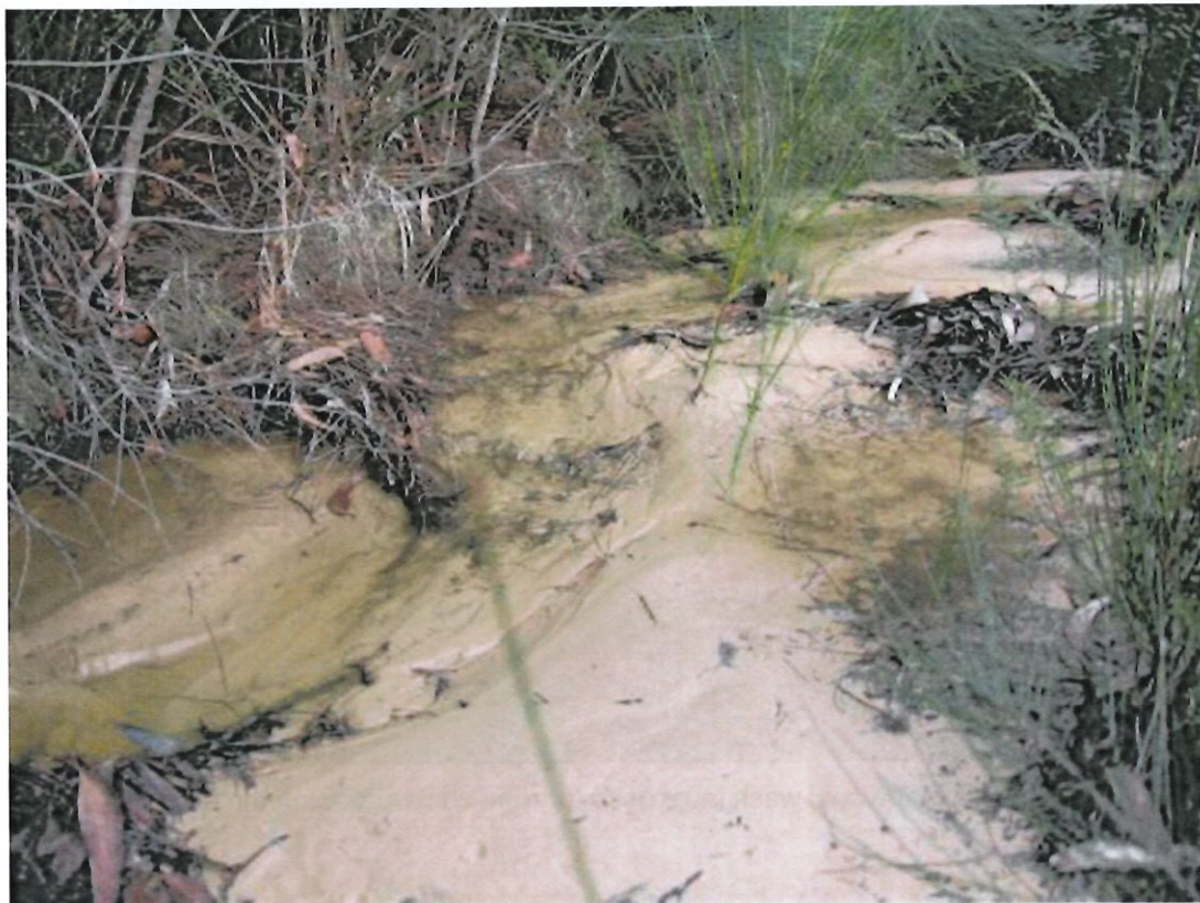
Figure 14- Close up picture of erosion pathway along the road shoulder, where coalwash was used.
