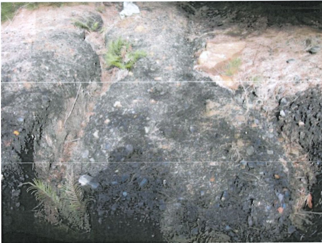
Figure 14- Close up picture of erosion pathway along the road shoulder, where coalwash was used.
